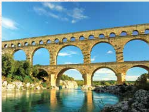
See the first-century Pont du Gard aqueduct, which was built with 55,550 tons of soft limestone blocks.
